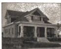
A No. 125-W IDEAL Boiler and 600 ft. of 3/4-in. AMERICAN Radiators, costing the owner $210, were used to heat this cottage. At this price the goods can be bought of any reputable, competent dealer. This did not include costs of labor, pipe, valves, freight, etc., which are extra, and vary according to climate and other conditions.
